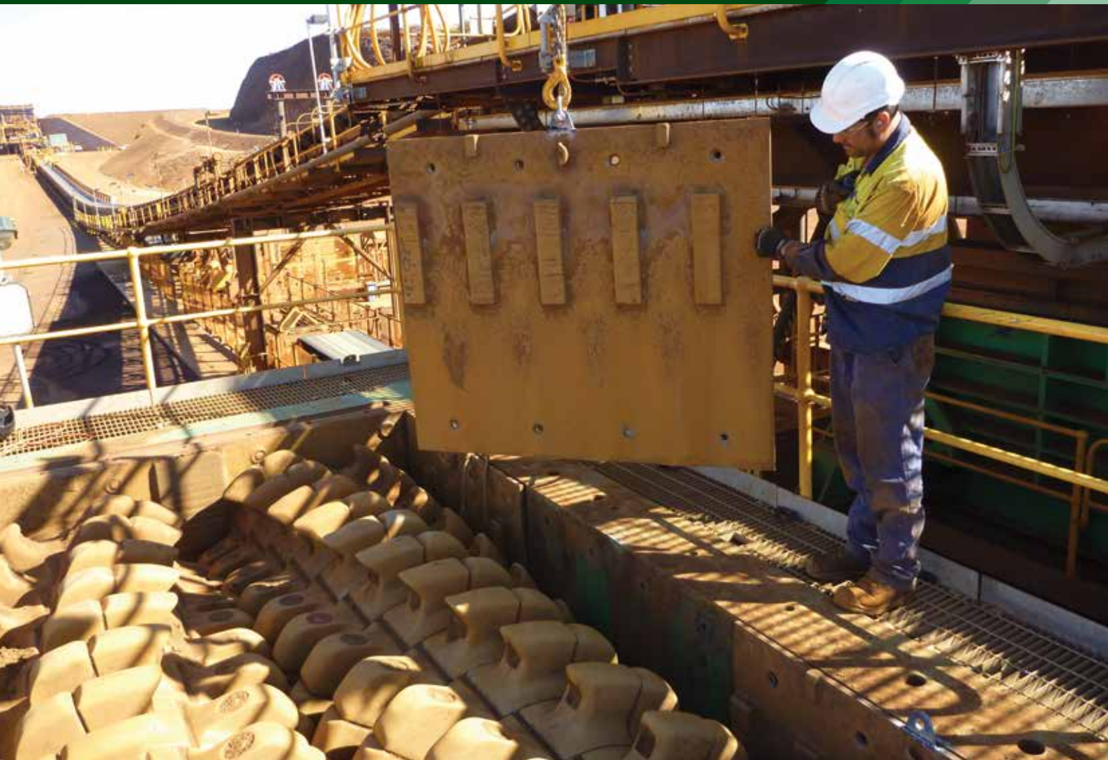
Mineral sizer repair work on-site in the Pilbara.
