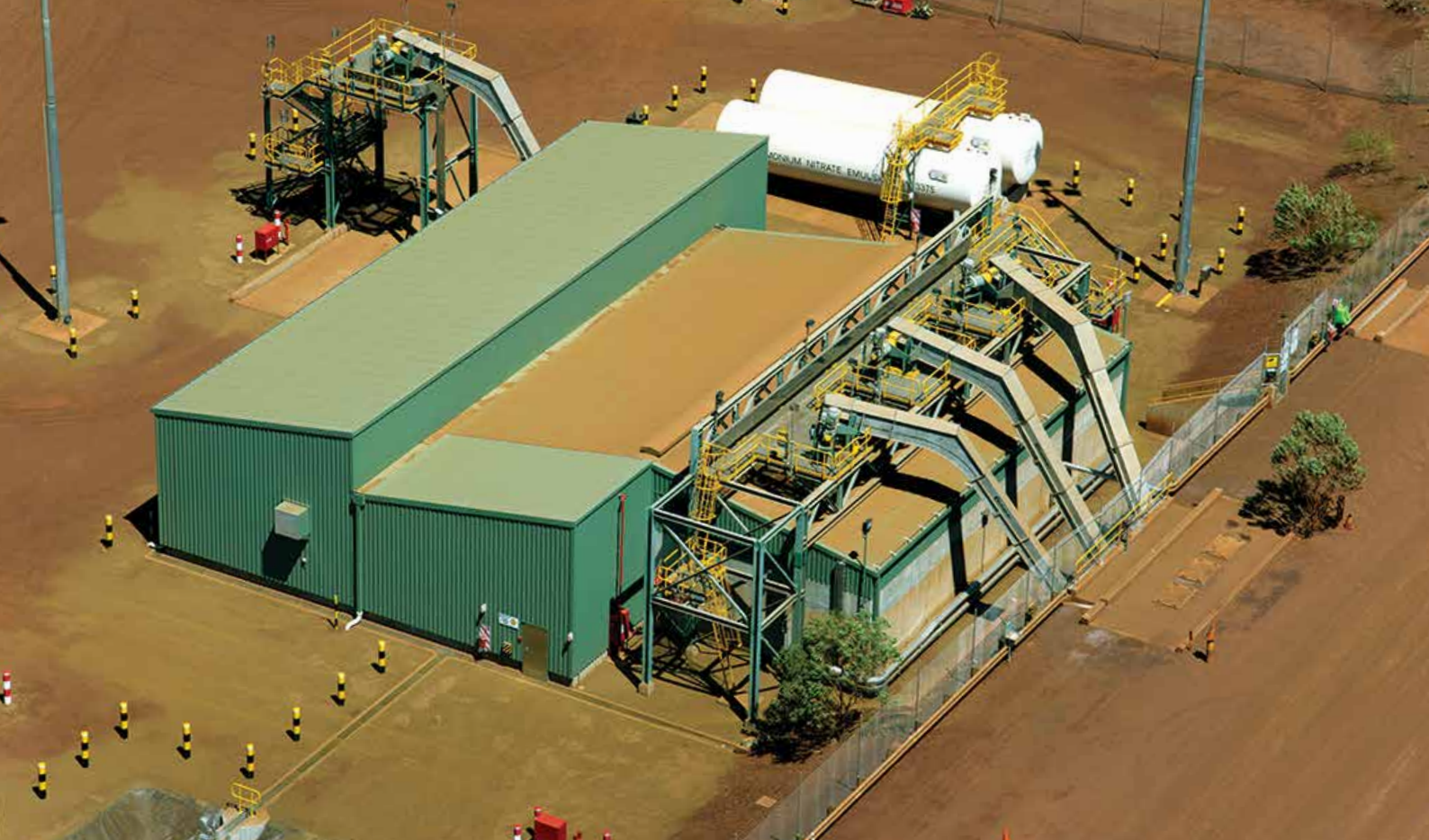
Ammonium nitrate prill intake and storage facility.
