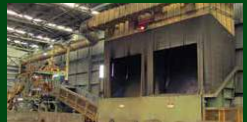
1500tph concentrate feeder at Bunbury Port.
